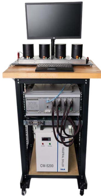
Figure 2: An example of a simple CellPod System. From top to bottom, items are: PC screen for the GUI, Quad showing four CellPods with insulating pods attached, PC keyboard, laptop control PC, Basytec cell cycler with 4x black cables, PSU (1U rack unit), coolant chiller (large white box). The PCAN is not visible in this image.
